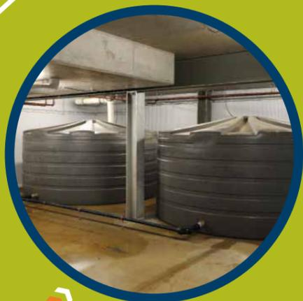
Water tanks capture roof water for use in the building for toilet flushing and landscape garden watering.
