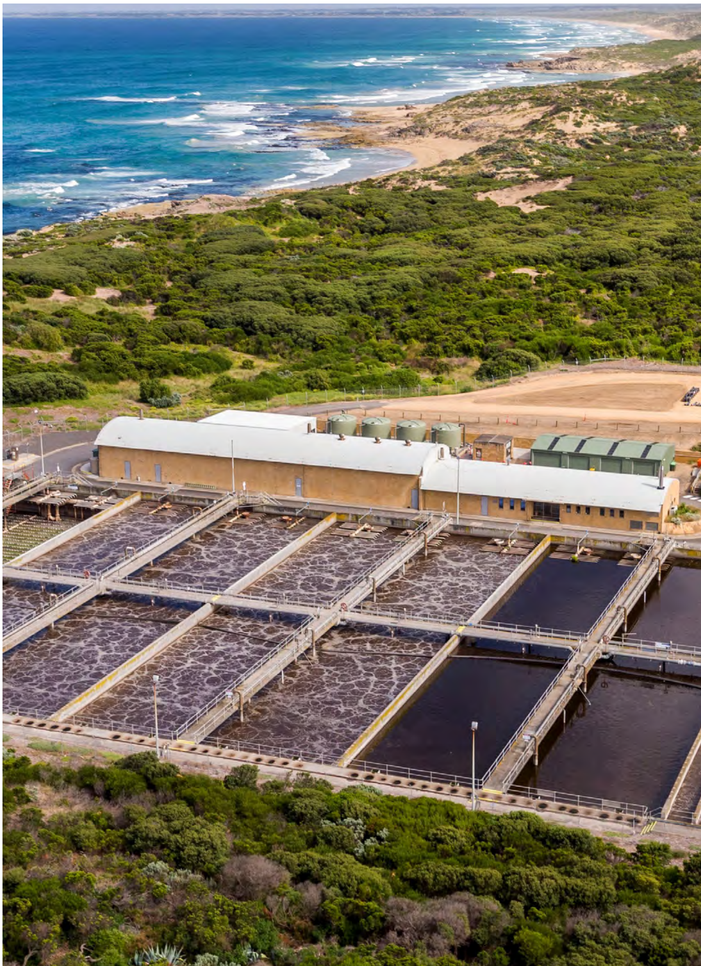
Warrnambool Sewage Treatment Plant
