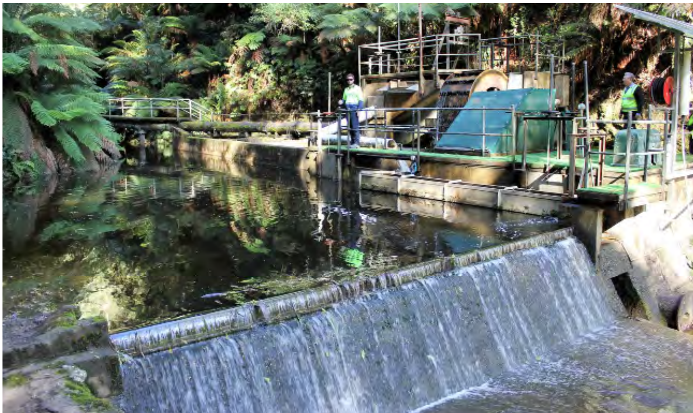
The West Arkins weir
