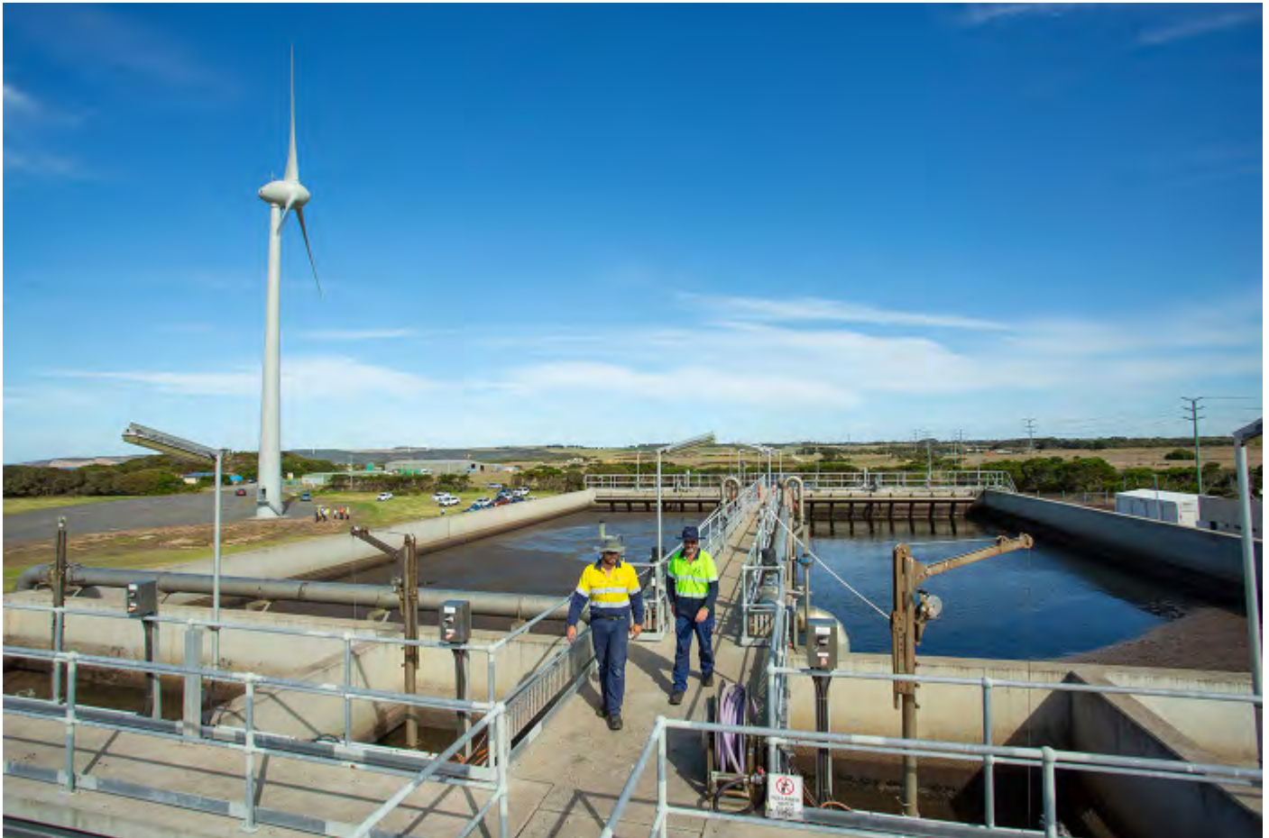
Portland Sewage Treatment Plant
