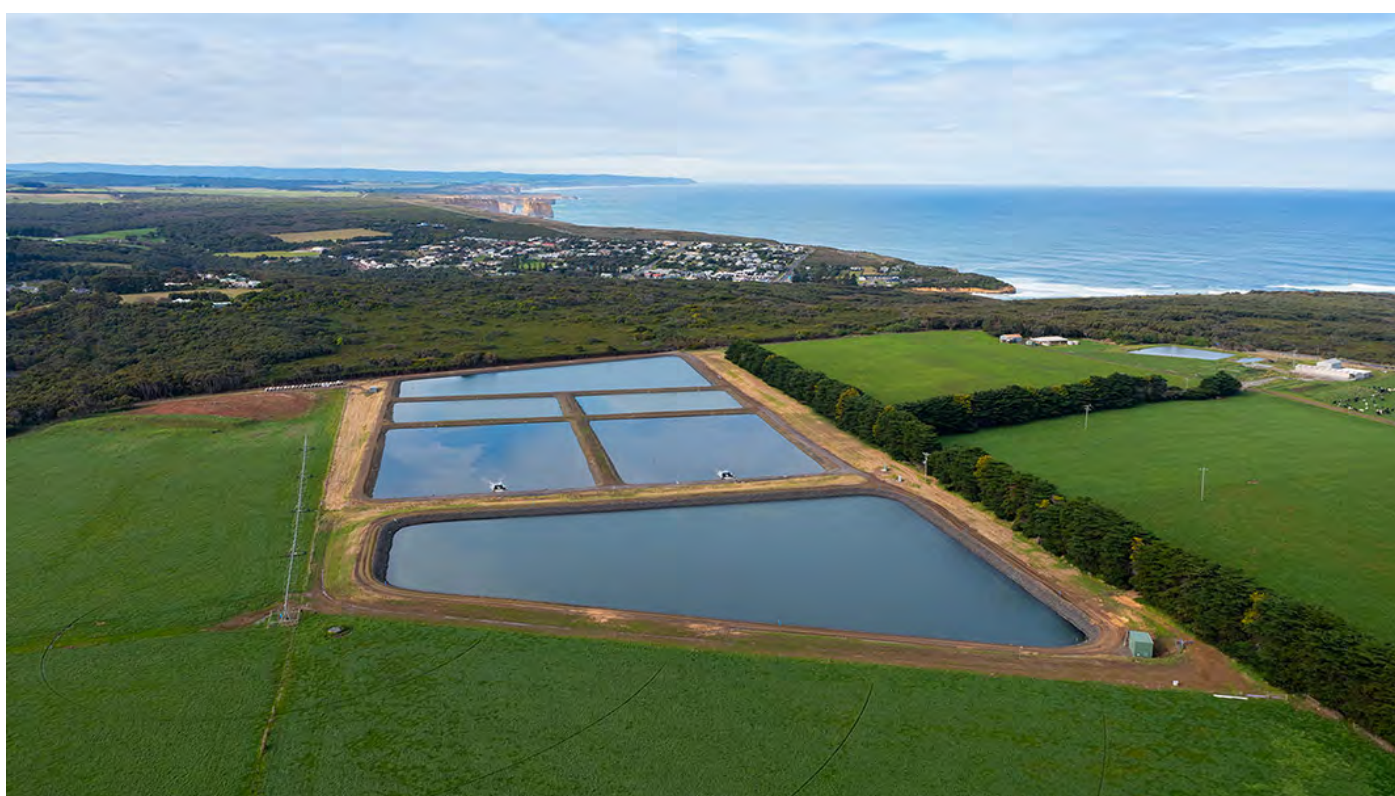
Port Campbell Sewage Treatment Plant
