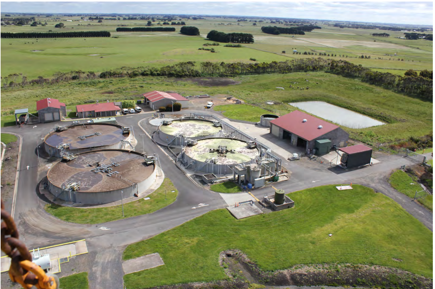
Port Fairy Sewage Treatment Plant
