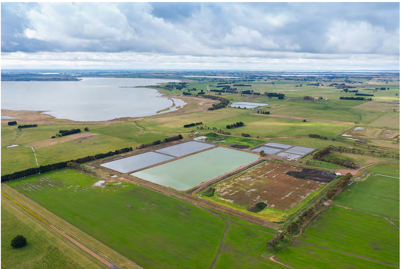
Camperdown Sewage Treatment Plant
