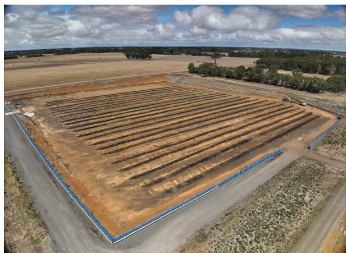
Biosolids drying area, Hamilton.
